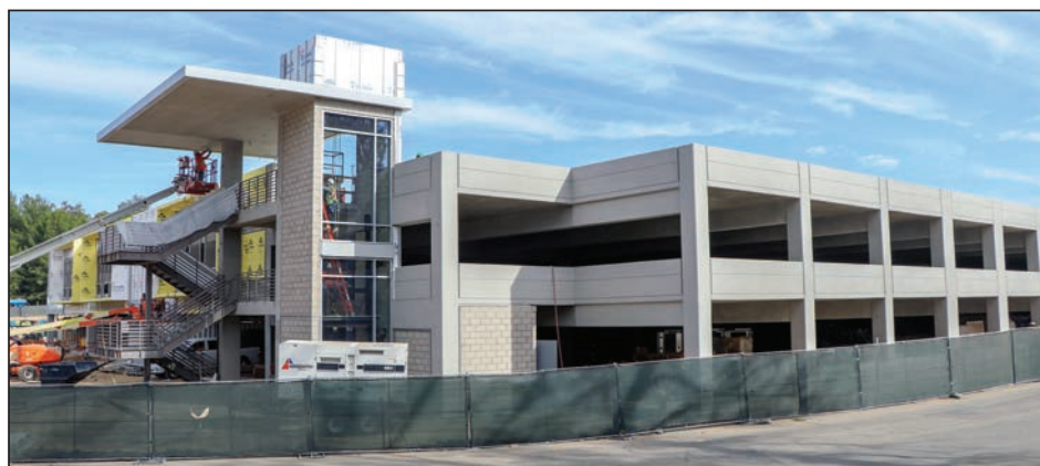
THE 1,659-SPACE PARKING STRUCTURE IS NEARING COMPLETION AT THE VALENCIA CAMPUS.
